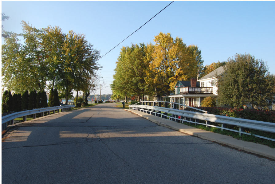
The inadequate approach to the bridge located on Edgewater Street, south of M-29, restricts vertical sight distances and creates a hazard to oncoming traffic.
